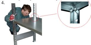
Place the bottom and topmost shelf between the two side frames on the rack mounts. If you are installing the rack alone, support one end of the rack against the wall to make the process
